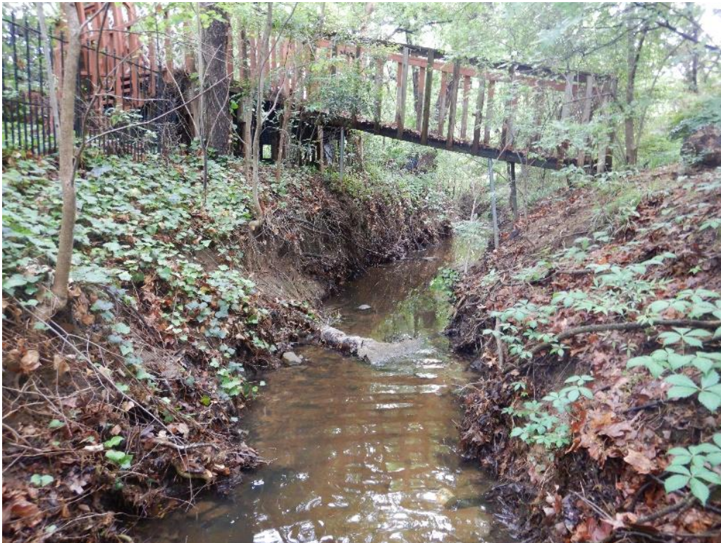
Station 9+00 - Looking downstream, this photo shows the representative conditions of the channel between station 6+00 and 10+00, also showing the concerns with Area of Concern #5
