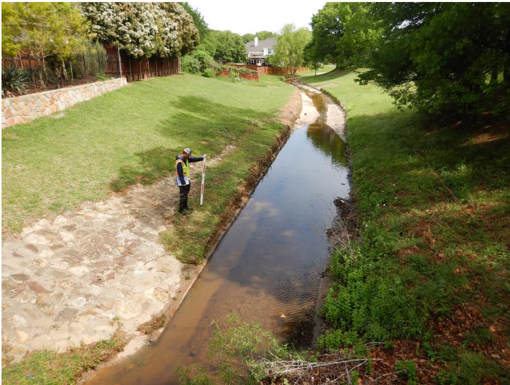
Downstream of Station 25+00 - Looking downstream from Cummings Drive at the concrete lined channel below the study area.
