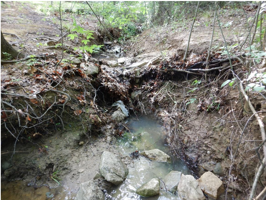
Station 14+50 - Looking upstream, this photo shows an approximately 3-foot head cut that may be migrating upstream into a stable section of channel ( Area of Concern #10 ).
