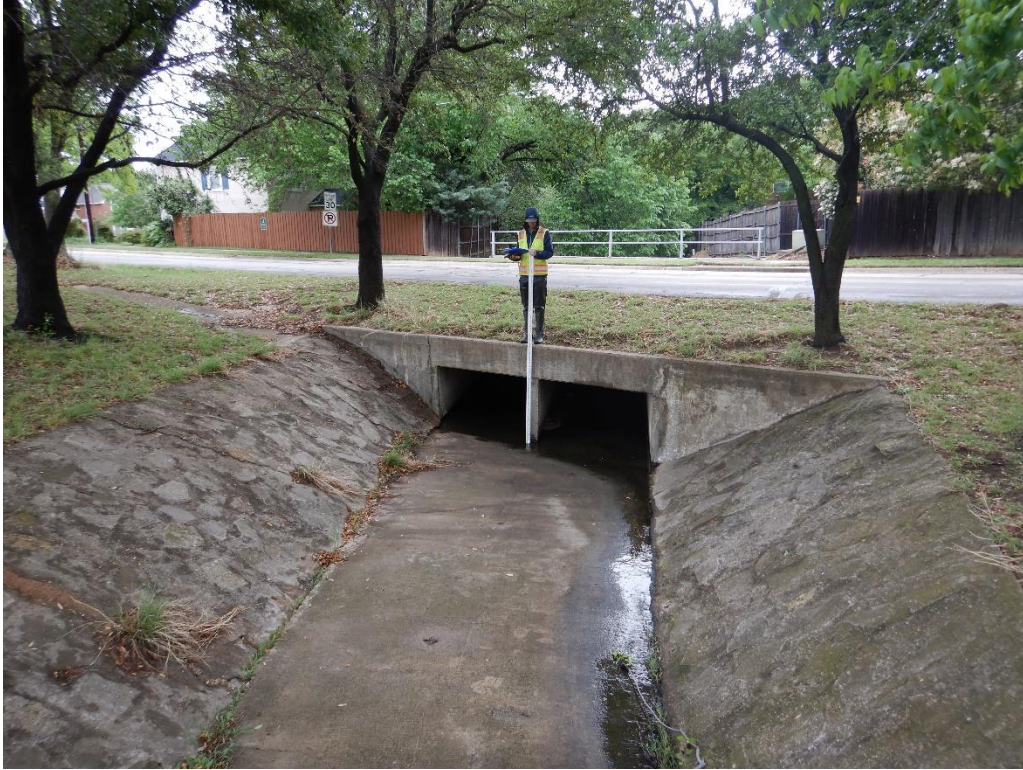
Upstream of Station 0+00 - Looking downstream at the Forest Drive culvert above the study area.
