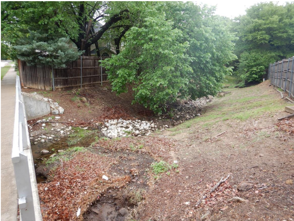
Station 0+00 -Looking downstream from Forest Drive.
