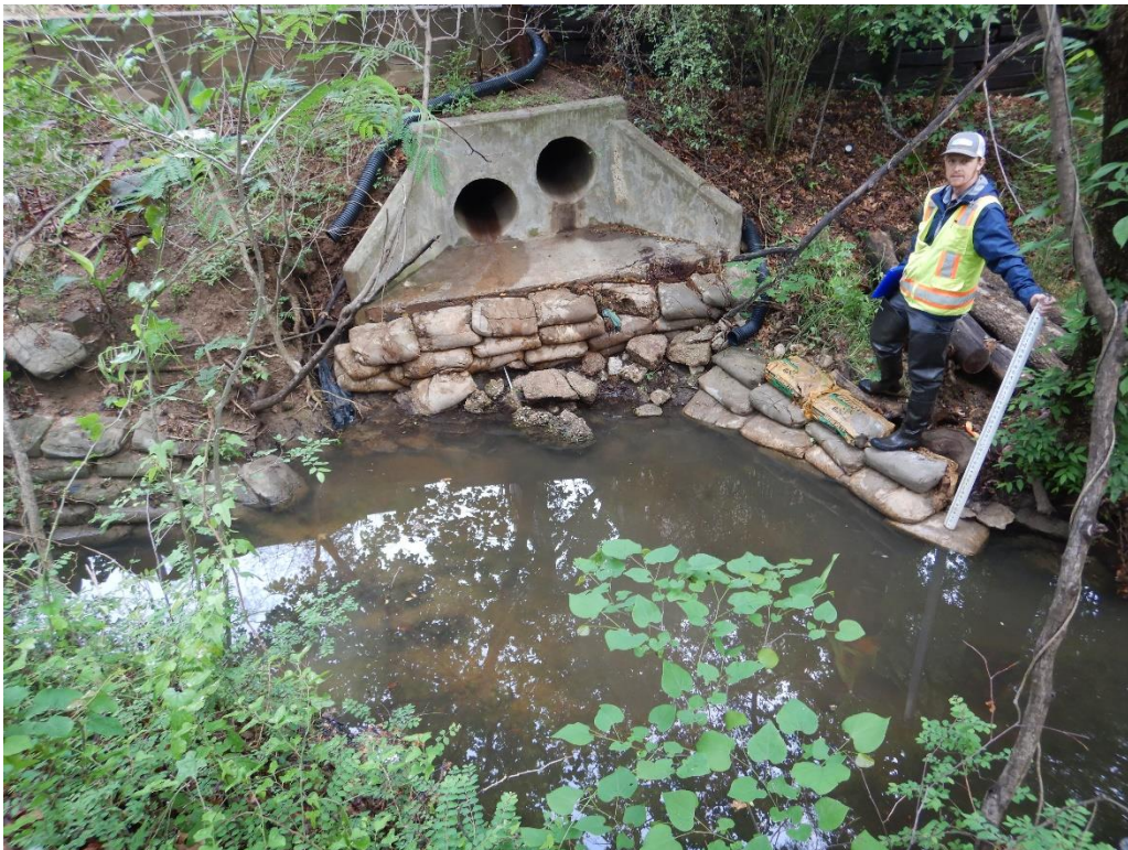
Station 13+00 - Looking at the left stream bank, this photo shows the condition of a stormwater outfall (Area of Concern #9).
