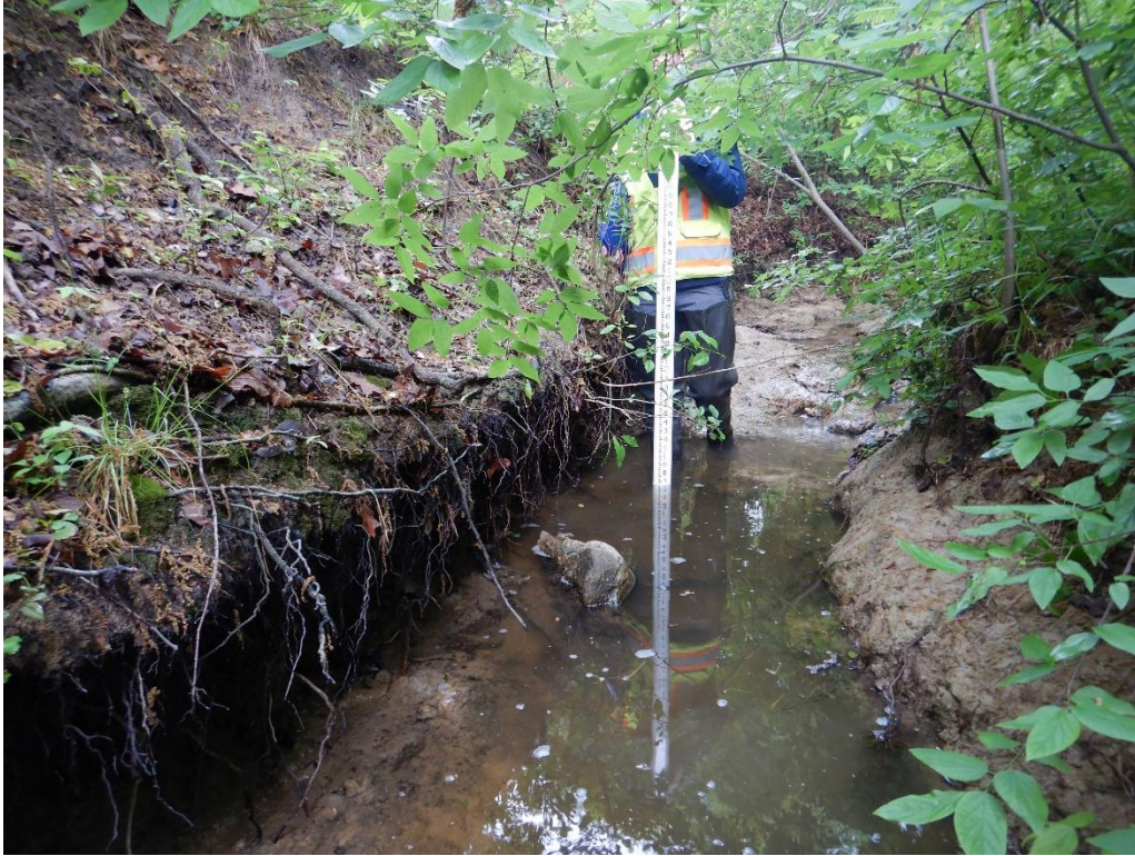
Station 6+00 - Looking upstream, this photo shows a representative example of a headcut propagating upstream.
