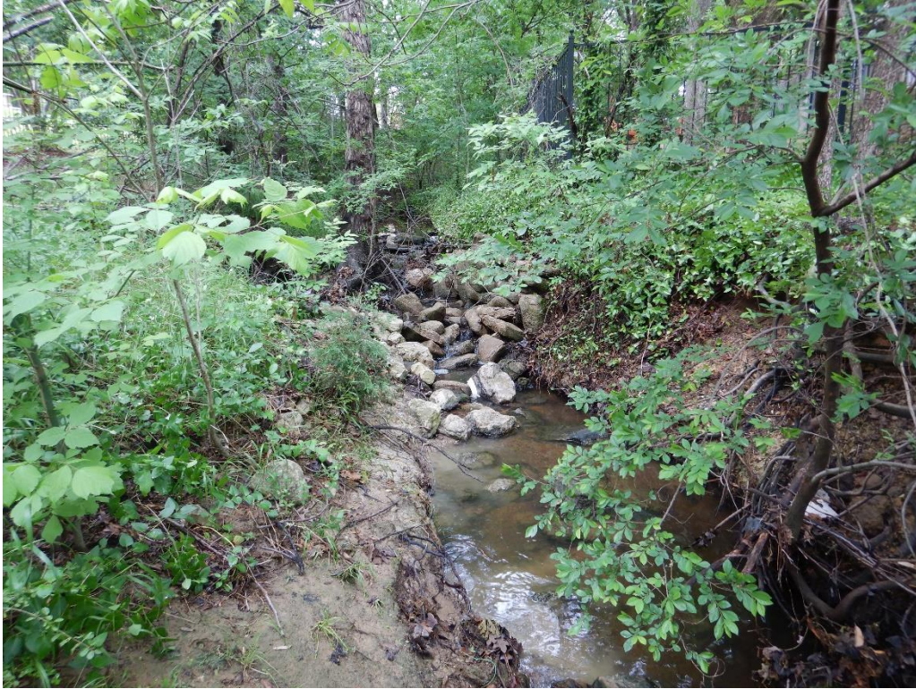
Station 10+75 - Looking upstream, this photo shows a headcut that is propagating upstream, and landowner attempts to prevent erosion impacts into back yards ( Area of Concern #8 ).
